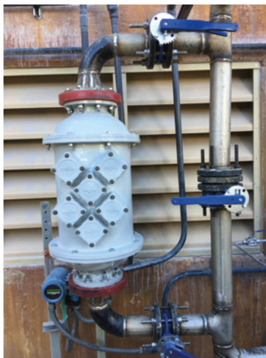
Arreglo by pass
